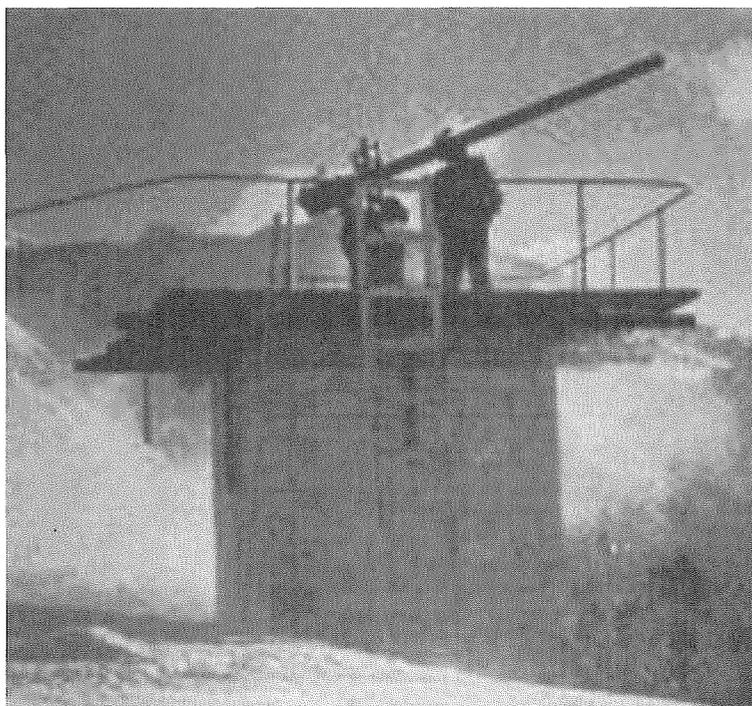
Figure 3 101mm Howitzer Recoilless Rifle used to artificially release avalanches
