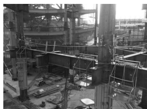
Photo 1.2 On-site construction of steel frames and beams
