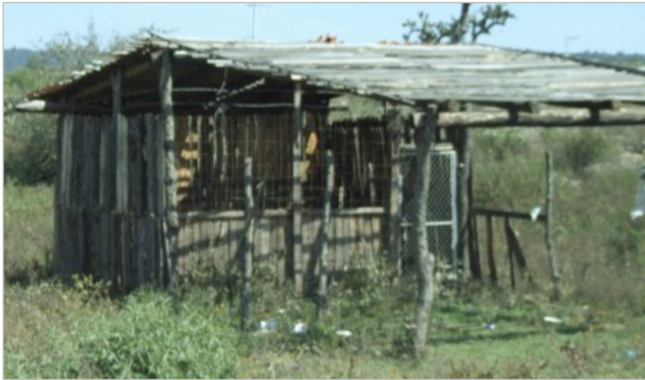
Figure 1: Building with base-to-ridge posts around Tapalpa in Jalisco State, Mexico, 2012
