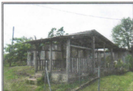
Figure 13: A structure with base-to-ridge posts in Cotton Tree, Belize (photo by the authors).
