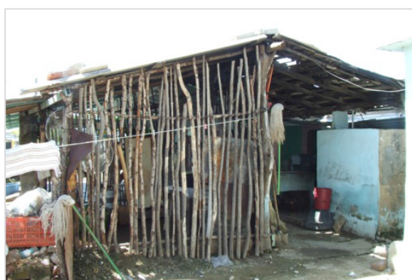
Figure 6 : Appearance of no. 20 with base-to-ridge posts Paredon, Mexico, 2013
