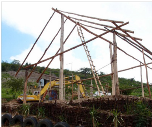
Figure 3: Appearance of no. 3 with base-to-ridge posts and its constructor peeling of eucalypti, Agua Salobrega, Guatemala, 2013
