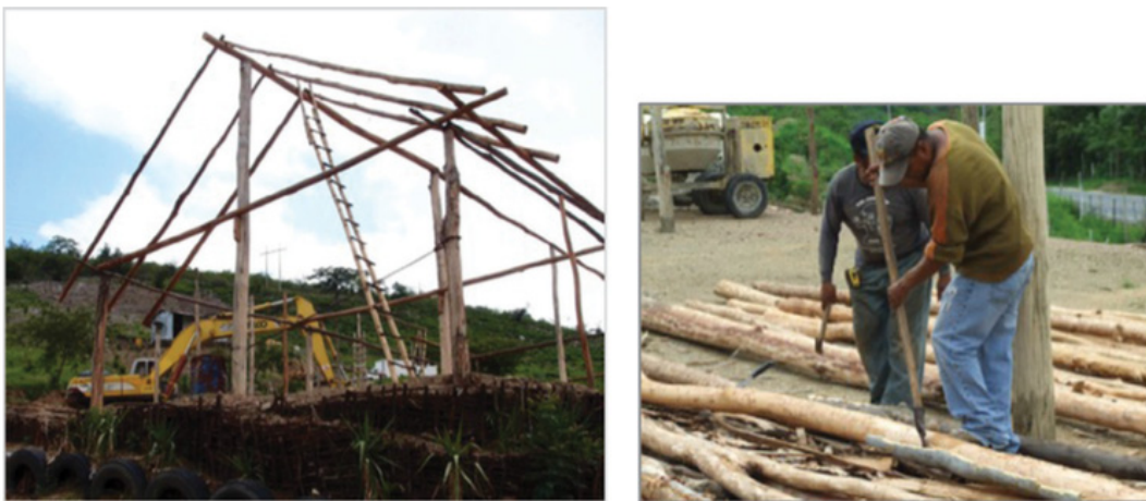
Figure 3: Appearance of no. 3 with base-to-ridge posts and its constructor peeling of eucalypti in Agua Salobrega, Guatemala, 2013.
