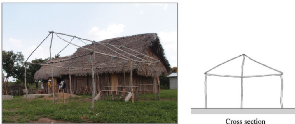
Figure 5: Appearance of no. 11 with base-to-ridge posts in Yemeri Grove, Belize, 2013.
