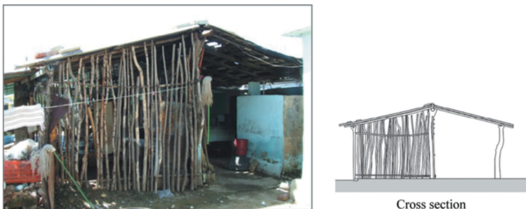
Figure 6: Appearance of no. 20 with base-to-ridge posts in Paredon, Mexico, 2013.
