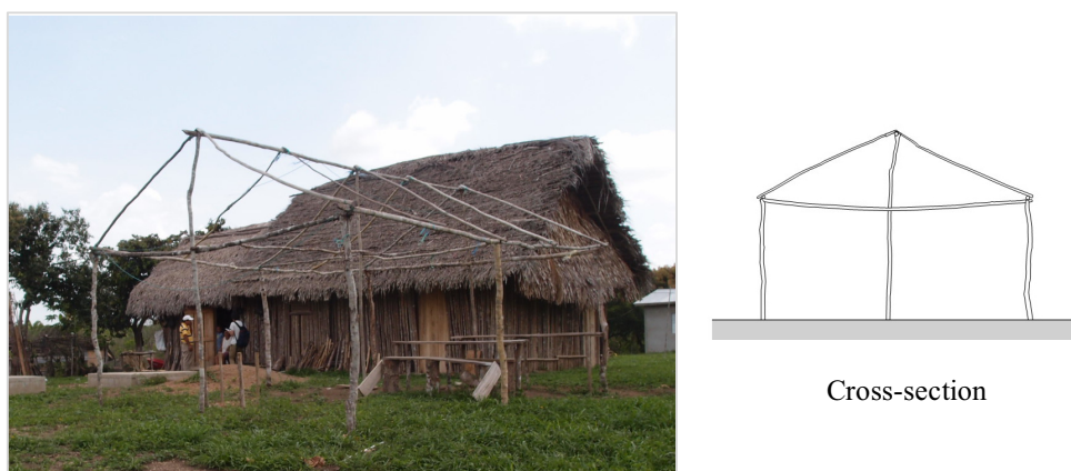
Figure 5: Appearance of no. 11 with base-to-ridge posts, Yemeri Grove, Belize, 2013
