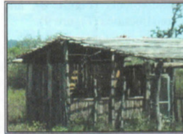
Figure 4: Buildings with base-to-ridge posts around Tapalpa 1, Mexico (photo taken by the authors).
