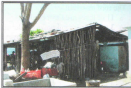
Figure 16: A structure with base-to-ridge posts in Paredón, Mexico (photo by the authors).
