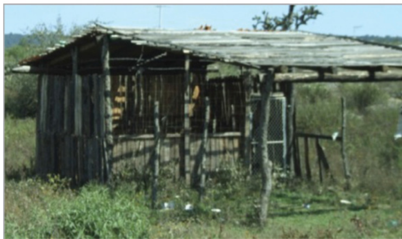
Figure 1: Building with base-to-ridge posts around Tapalpa in Jalisco State, Mexico, 2012.
