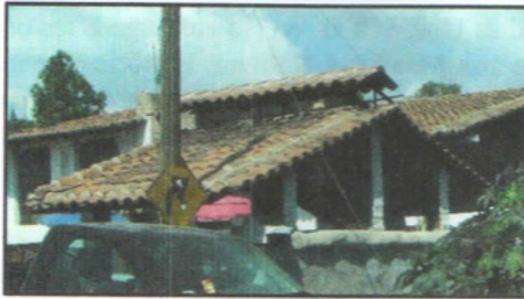
Figure 5: Buildings with base-to-ridge posts around Tapalpa 2, Mexico (photo by the authors).
