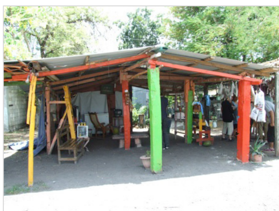
Figure 4: Appearance of no. 18 with base-to-ridge posts, Xalapa, Mexico, 2013
