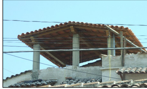
图6 Buildings with base-to-ridge posts around Tapalpa 3, Mexico, photo by the authors.
